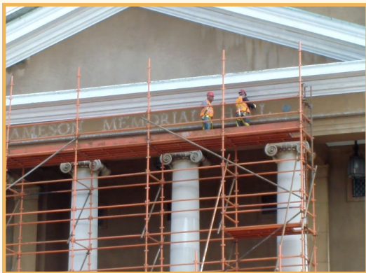
Image 19: De-lettering of Jameson Memorial Hall. University of Cape Town. UCT Communications / Newsroom.
